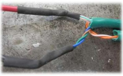
two soldered junctions and shrink as shown in the photo above.
